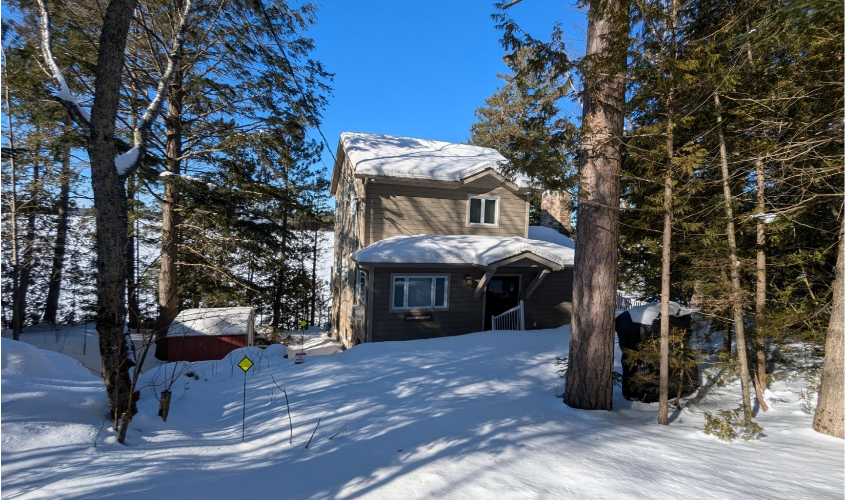
Figure 1 Existing dwelling from rear facing north.
