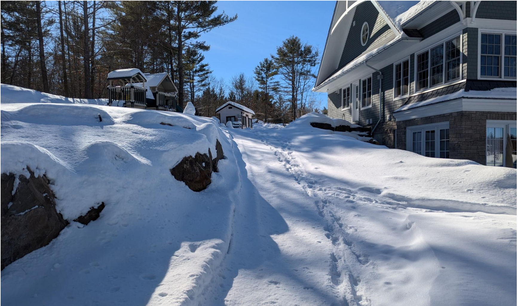
Figure 1 Subject property facing south from water yard.
